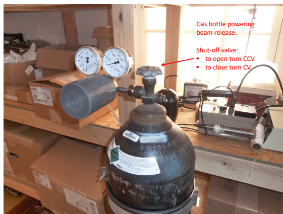
Figure 10.3: Gas bottle powering the pneumatic cylinder used to release the beam.
