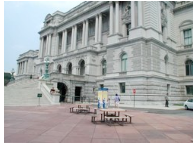
Library of Congress, Jefferson building
